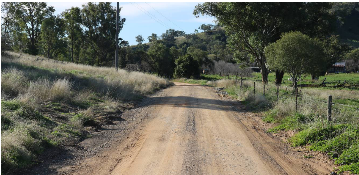
Photograph 5 – Black Gully Road.
