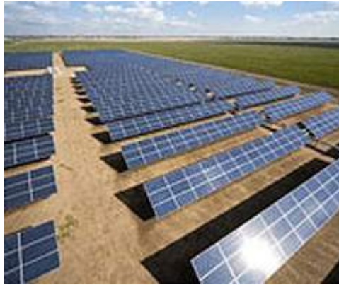
Photo 2: Example of solar farm panels
