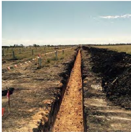
Photo 4: Example of underground cable trench with bedding sand installed.
